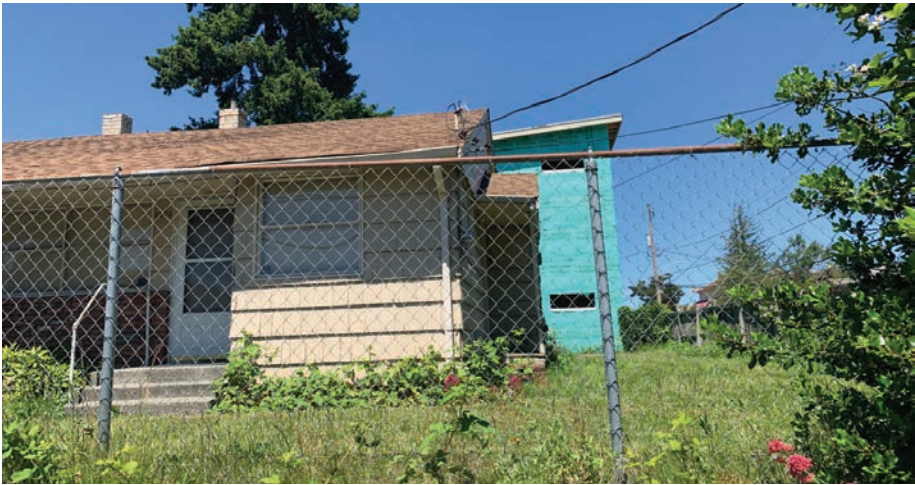
D SOUTH VIEW FROM SOUTH MYRTLE STREET
