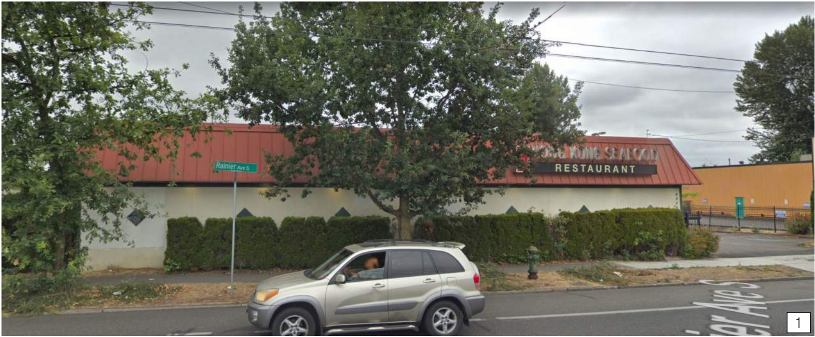
EXISTING BUILDING - VIEW TO NORTH
