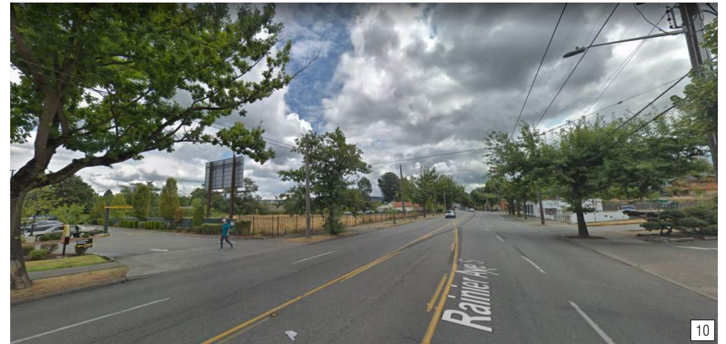
RAINIER AVENUE SOUTH - VIEW TO NORTHEAST
