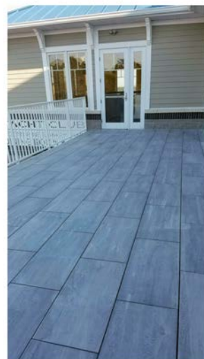
ROOF TOP DECK Deckstone Porcelain Pavers
