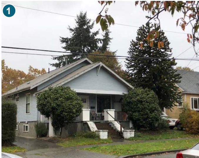
OLDER HOMES NEAR SITE, TYPICAL OF AREA
