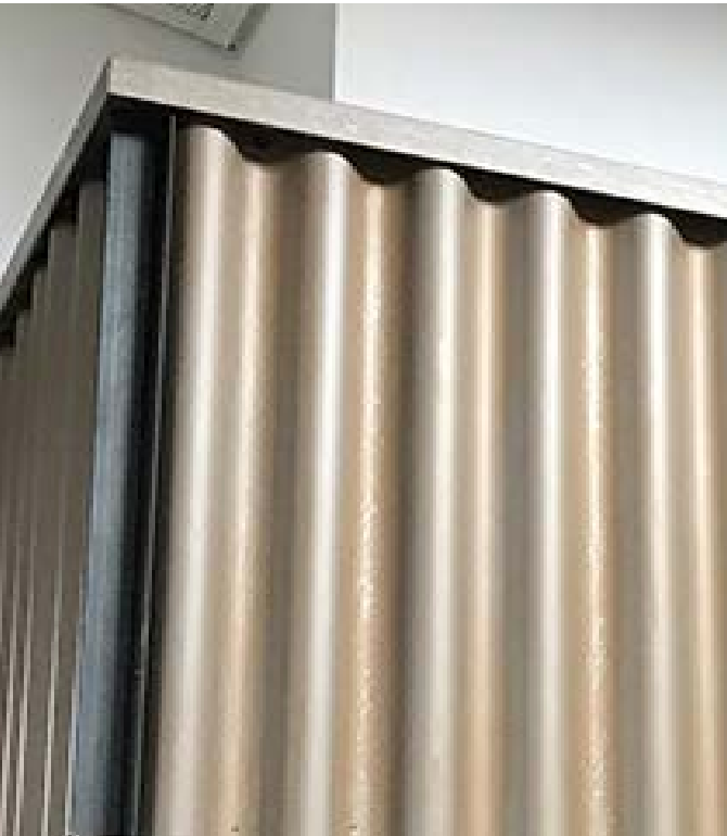
MP CORRUGATED METAL PANEL WESTERN STATES ROOFING STREAKED GALVANIZED RUST
