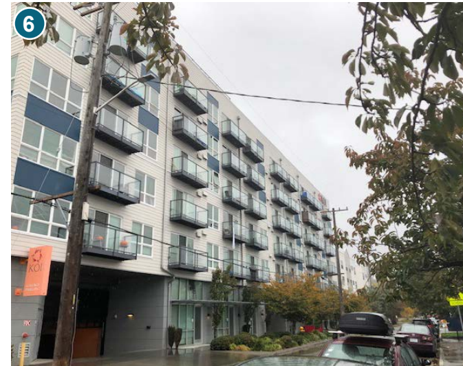
KOI - NW 54TH FACADE 6-STORY MIXED-USE RESIDENTIAL
