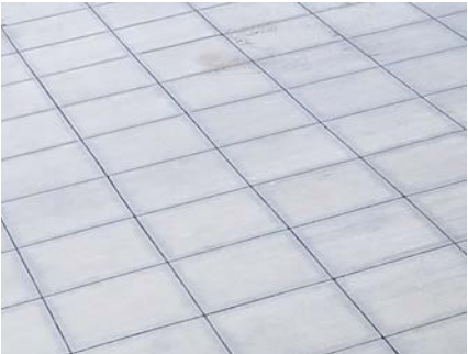
Scored Concrete; Sawcut Finish
