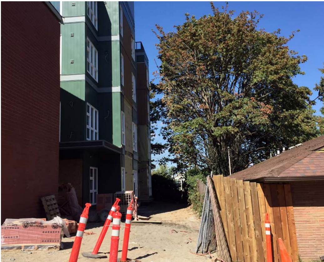
NEIGHBORING CONSTRUCTION TO THE WEST
