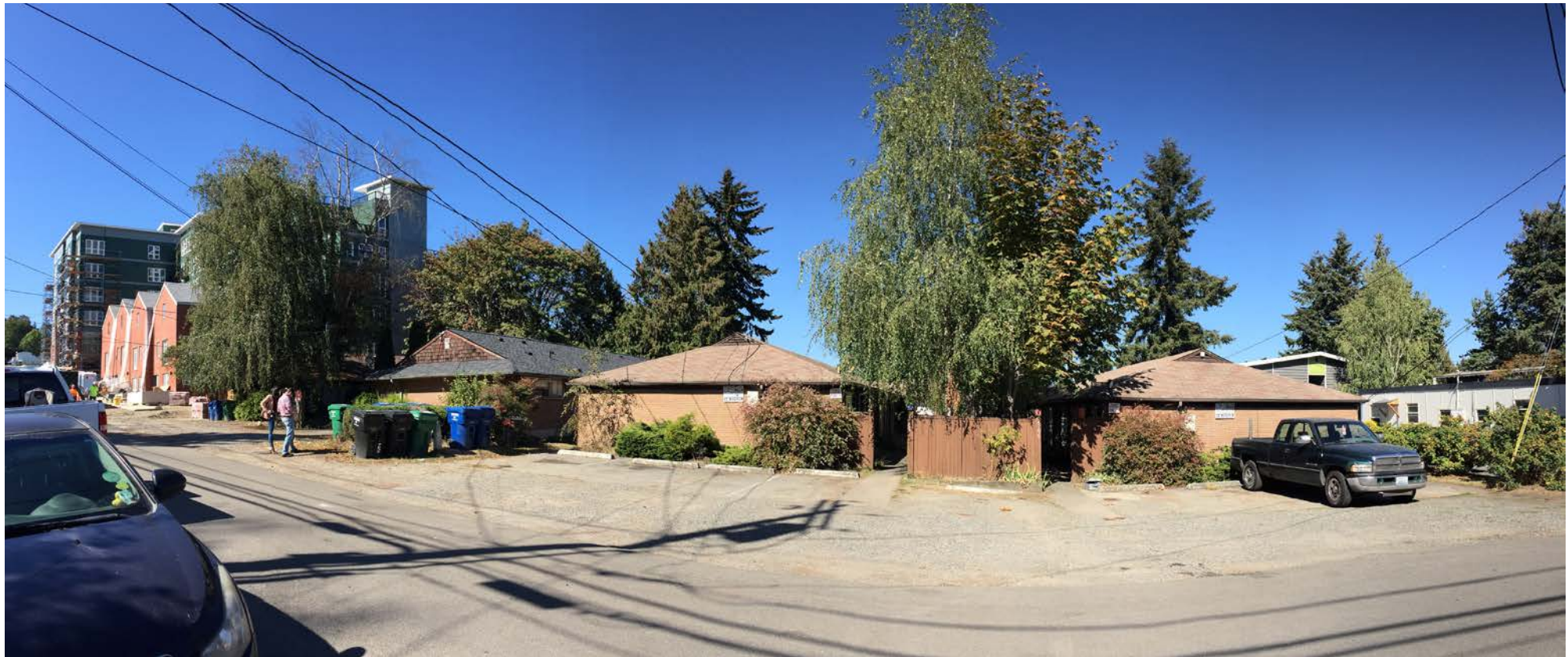
SITE FACING NORTH FROM 85TH AVE
