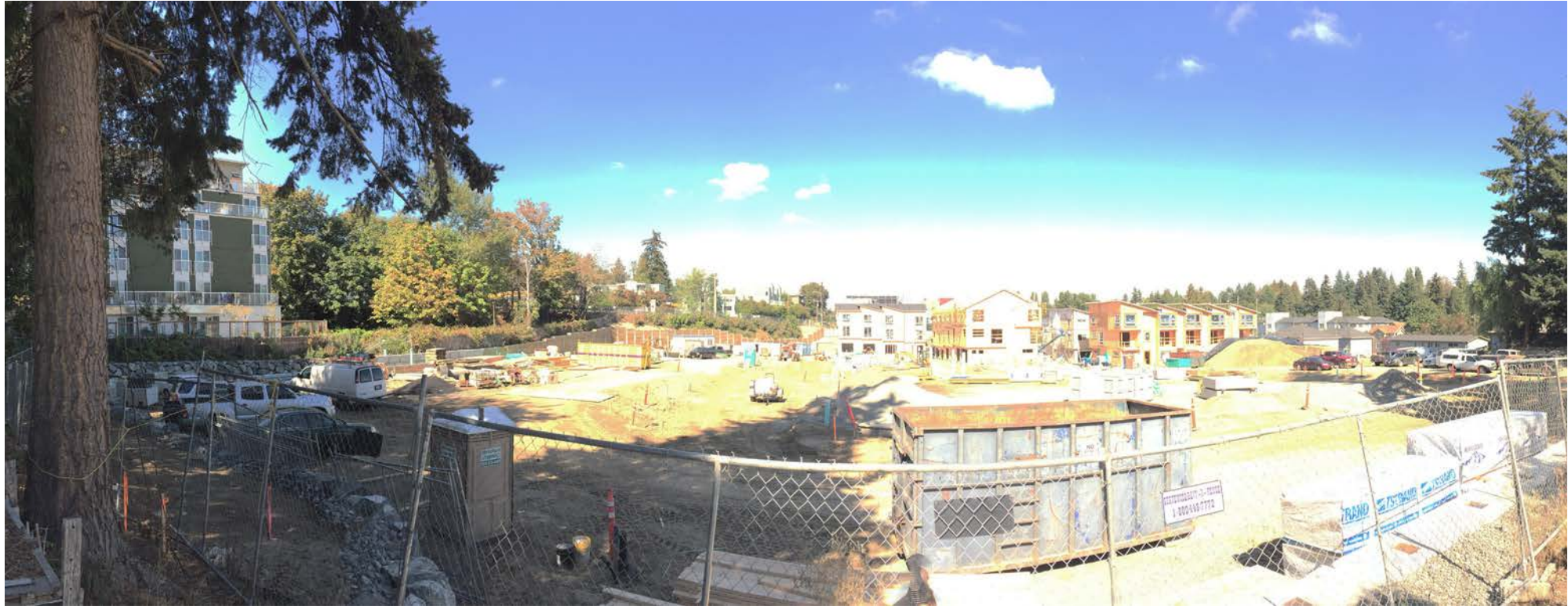
NEIGHBORING CONSTRUCTION TO THE NORTH
