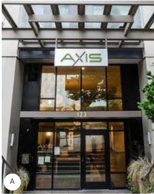
12” High stainless steel sign attached to underside of canopy.
