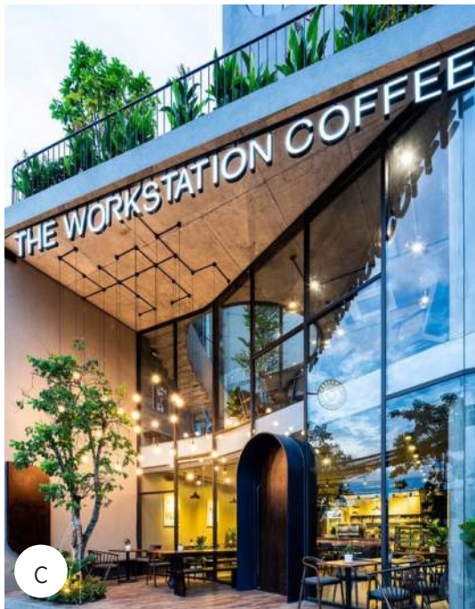
12” High stainless steel letters attached to underside of canopy
