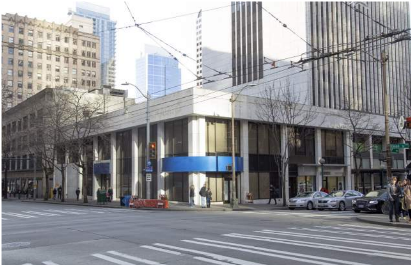
Existing Building on Site
