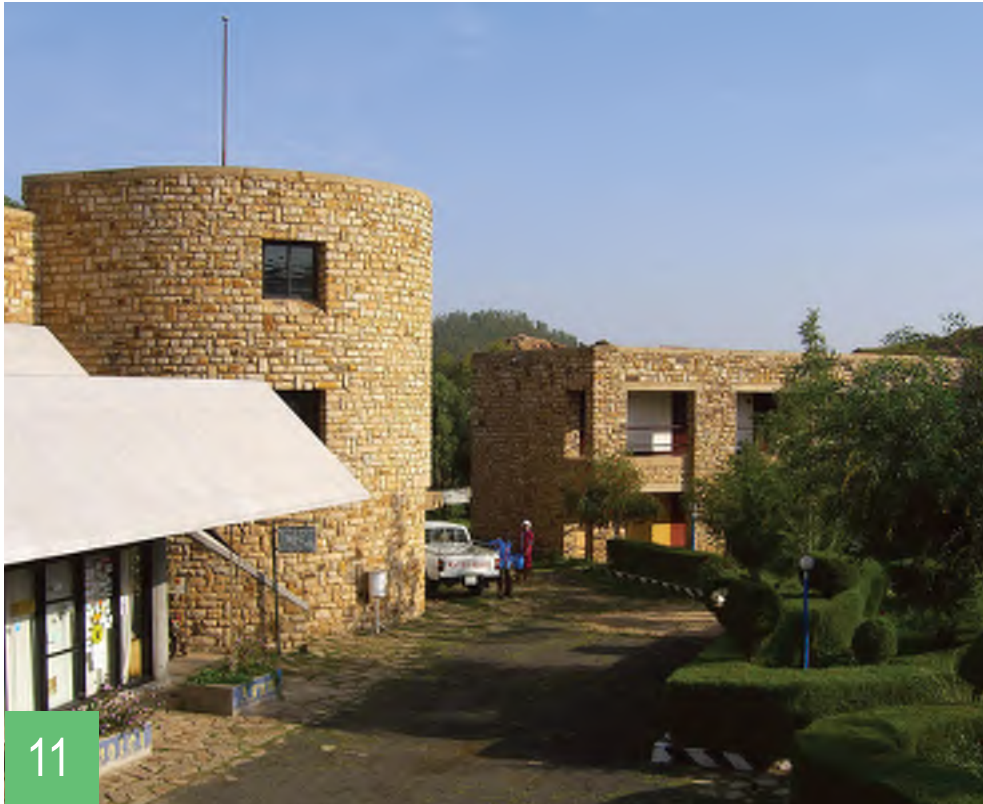
11 SAMPLE OF RECENT CONSTRUCTION - Masonry coursing and color variation - Reference to vernacular shapes
