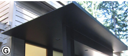
THIN PROFILE BENT STEEL AWNING (FINISHED TO MATCH PLYGEM BRONZE)
