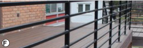
F HORIZONTAL RAILING (FINISHED TO MATCH PLYGEM BRONZE)
