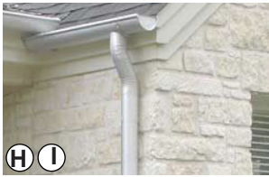
DOWNSPOUT/SCUPPER (WHITE FLOUR)
