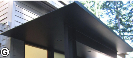
G THIN PROFILE BENT STEEL AWNING (FINISHED TO MATCH PLYGEM BRONZE)
