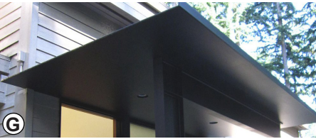
THIN PROFILE BENT STEEL AWNING (FINISHED TO MATCH PLYGEM BRONZE)
