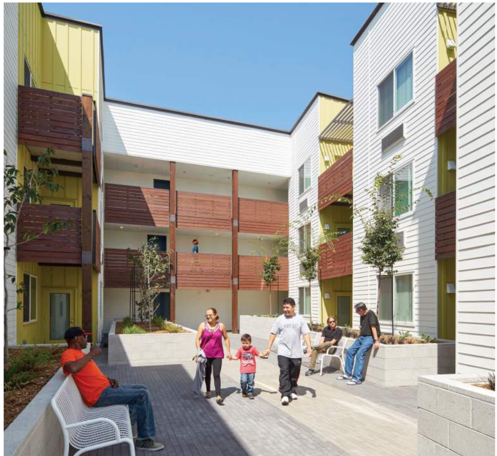
DC3-B-4: Exterior walkways connect to courtyards Onizuka Crossing Family Housing, David Baker Architects
