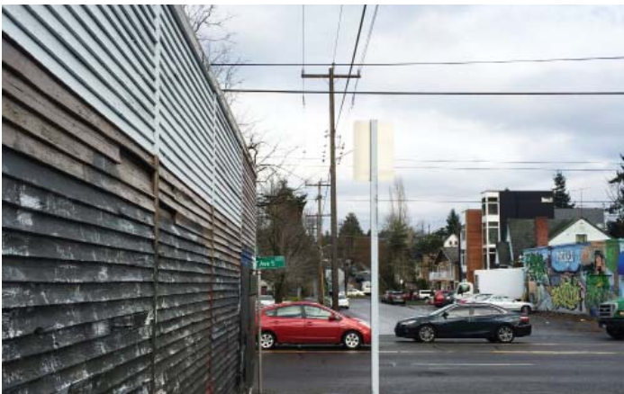
9 VIEW OF SE CORNER FROM S. BYRON ST.
