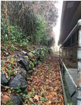
6 VIEW ALONG NORTH PROPERTY LINE LOOKING EAST
