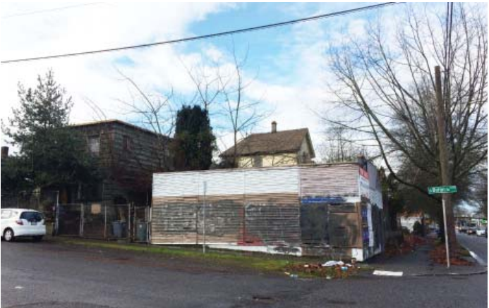
1 VIEW FROM SE CORNER-INTERSECTION OF RAINIER AVE S. AND S. BYRON ST.
