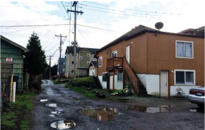
9 VIEW OF SW CORNER FROM ALLEY
