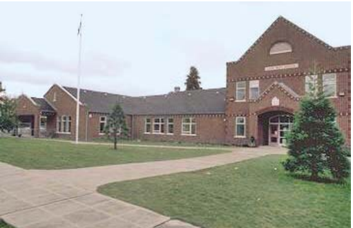
2 JOHN MUIR ELEMENTARY SCHOOL 0.3 Mile from Project Site
