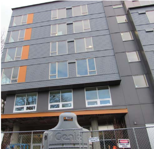
4 3501 RAINIER AVE S - UNDER CONSTRUCTION
