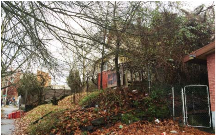
7 EXISTING SINGLE FAMILY RESIDENCE AND ROCKERY AT NORTH PROPERTY LINE
