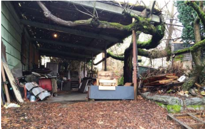
1 VIEWS OF EXISTING SINGLE FAMILY RESIDENCE FROM S. BYRON ST.
