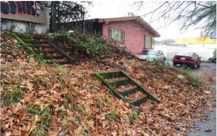
4 EXISTING SITE STAIRS AND SLOPE TOWARDS RAINIER AVE S.
