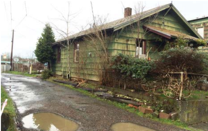
4 VIEW OF ALLEY FROM SW CORNER
