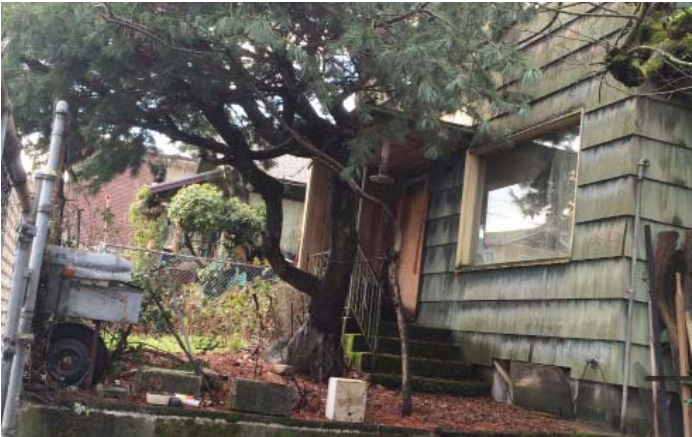
2 VIEWS OF EXISTING SINGLE FAMILY RESIDENCE FROM S. BYRON ST.
