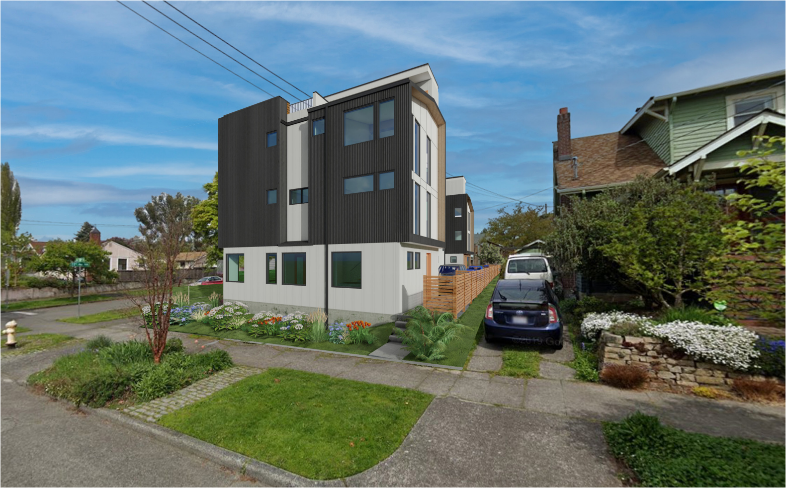
2. APPROACH FROM SE ON NW 58TH ST
