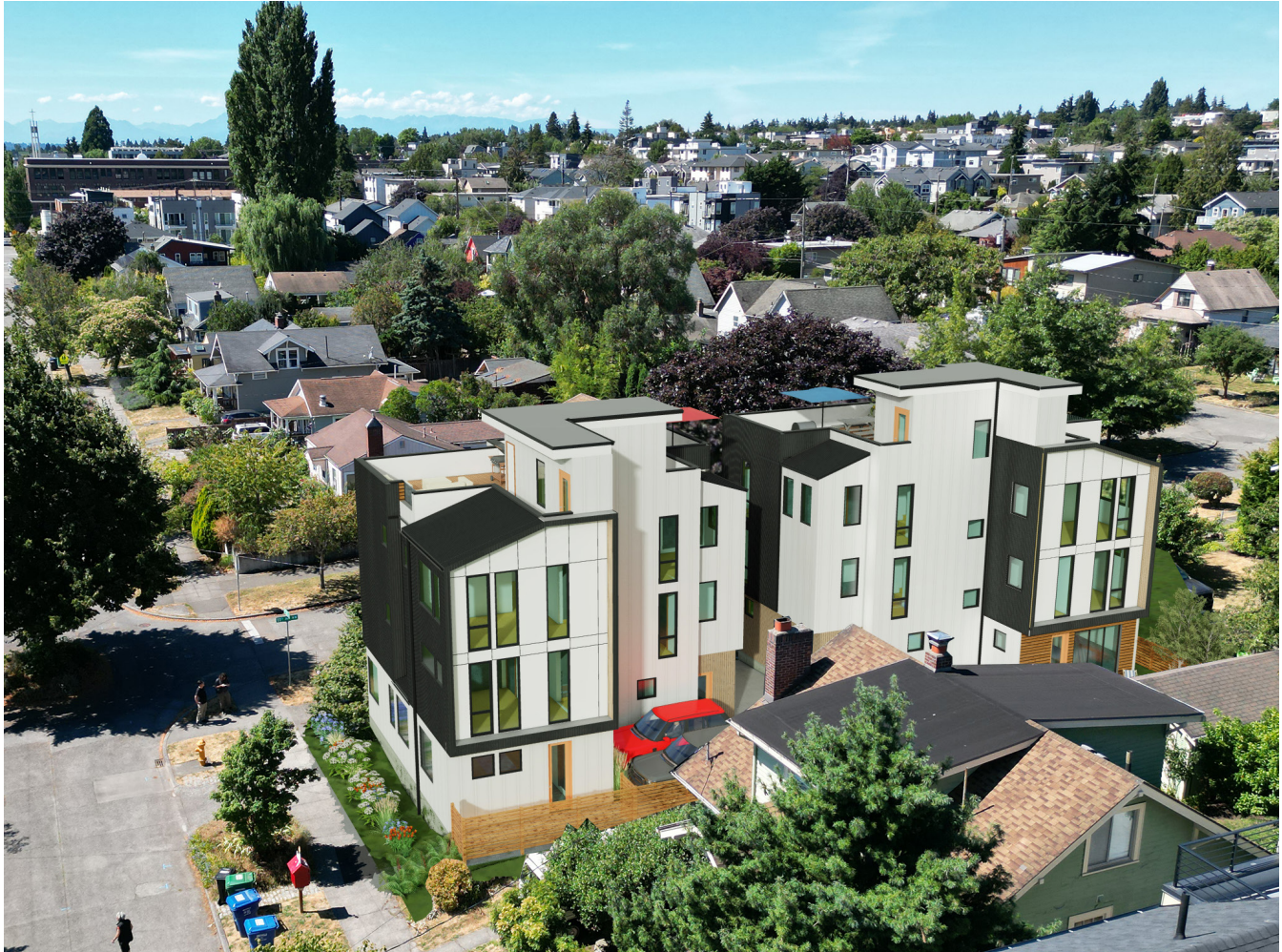
2. AERIAL VIEW REAR FACADE
