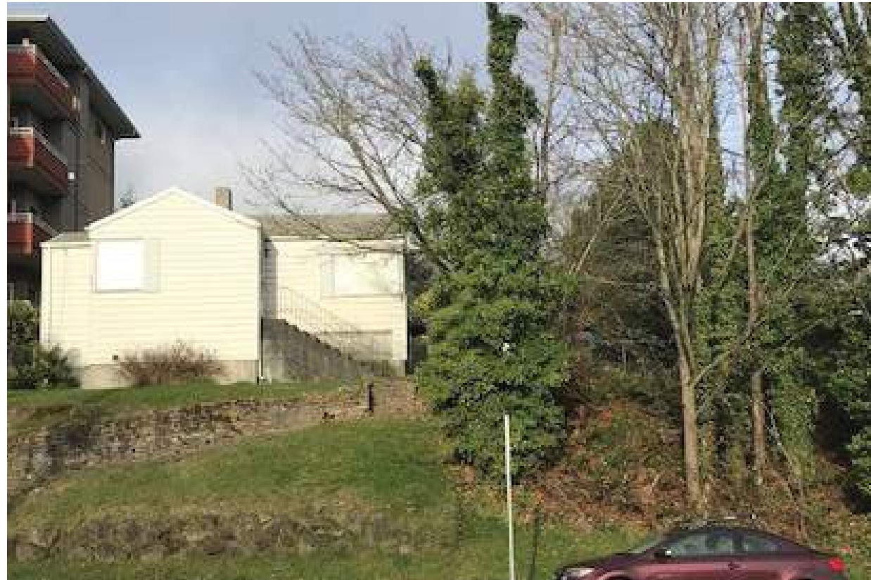
NEIGHBORING STRUCTURE TO THE SOUTH.
