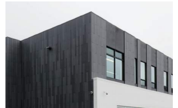
VERTICALLY ORIENTED FIBER CEMENT SIDING
