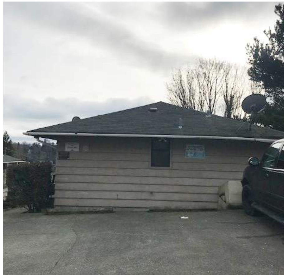
LOOKING EAST TOWARDS SITE FROM ALLEY.
