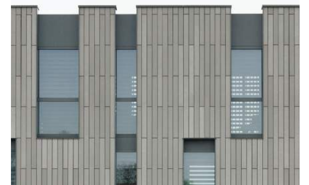
PANEL INFILL AT WINDOW ALIGNMENT
