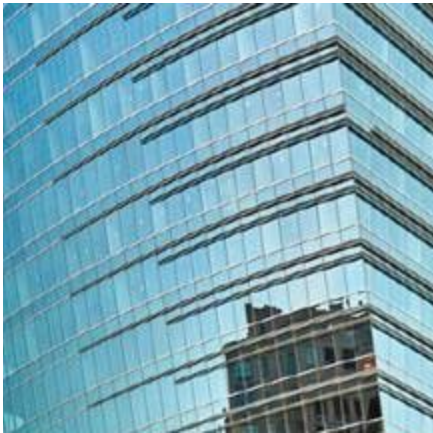
South Tower Manufacturer: Guardian Glass System: Window Wall Glass: SNR 43 on Clear (#2) Harmonizing Spandrel Color: Subdued Gray (#4) Example: McKinney and Olive Mixed-Use Facility Location: Dallas, TX
