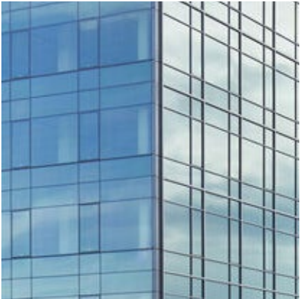
North Tower Manufacturer: Guardian Glass System: Window Wall Glass: SNX 62/27 on Clear (1" double-glazing) Harmonizing Spandrel Color: Knoxville Gray Example: Southport Office Complex Location: Renton, WA
