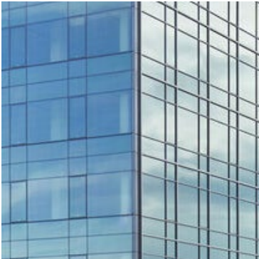
GL-01 Window Wall Glazing Manufacturer: Guardian Glass Glass: SNX 62/27 on Clear (1" double-glazing)
