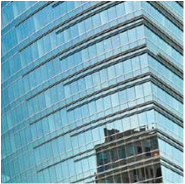
GL-05 Window Wall Glazing Manufacturer: Guardian Glass Glass: SNR 43 on Clear (#2)
