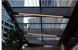
Luminous Ceiling -Back lit glass ceiling over the drop off creates a bright, safe alley-side presence.
