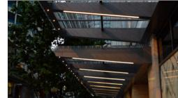
2 Soffit Downlights -Round downlights illuminate from soffits in front of the garage, loading dock, and exit doors.
