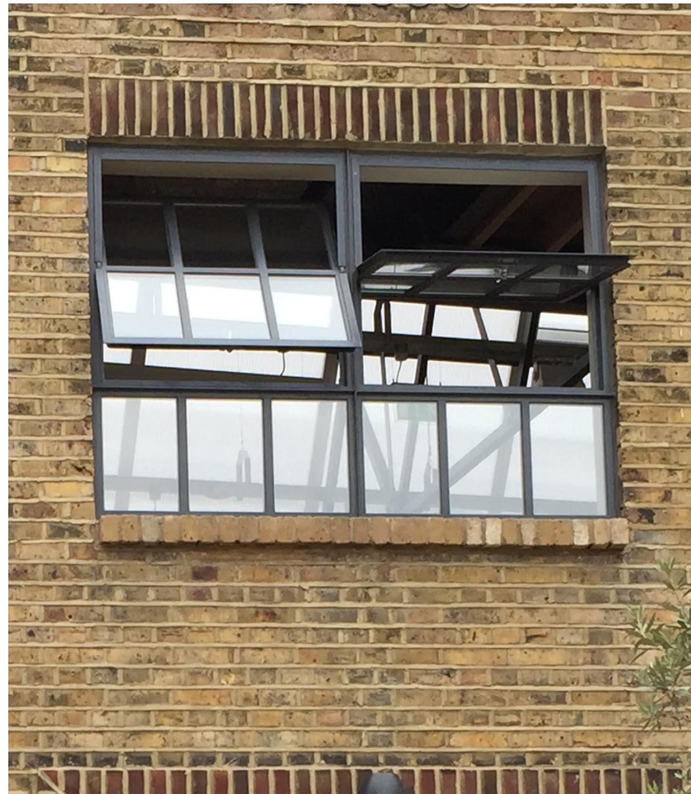
Image of Steel Pivot Window System
