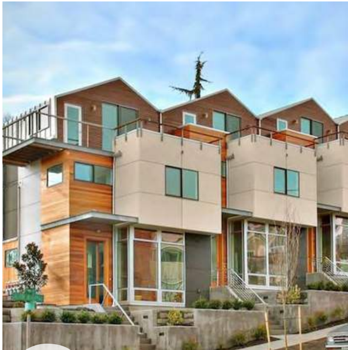
5. High density results in smaller living situations; contemporary materials and massing strategies are prevalent.
