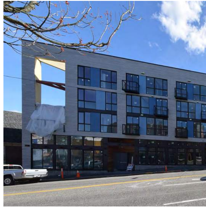
2. Local buildings use contemporary materials such as wood paneling, metal and synthetic paneling, such as the fiber reinforced concrete "oko" paneling shown in the building across the street.
