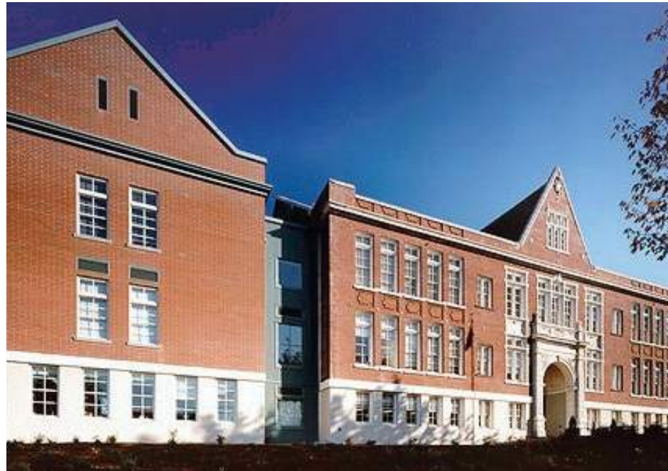
1 - GREENWOOD ELEMENTARY SCHOOL
