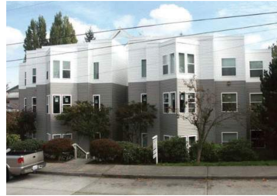
3 - CROWN HILL COURT APARTMENTS
