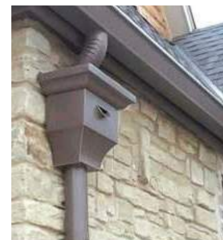
10) PREFINISHED COPING, GUTTERS, DOWNSPOUTS
