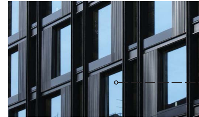
depth and detail of facade
