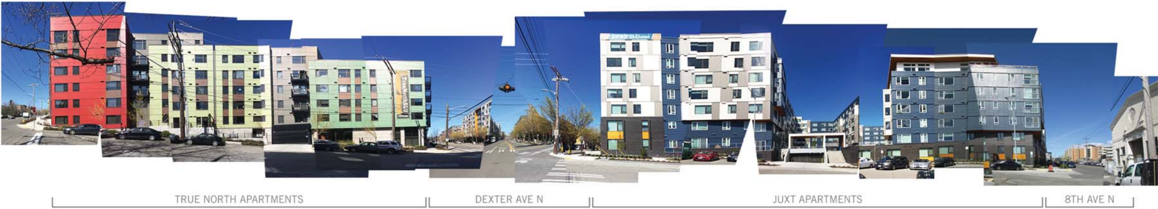
2 STREETScape ALONG VALLEY ST LOOKING NORTH
