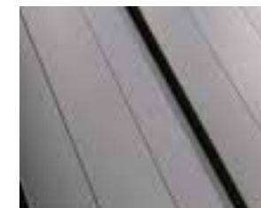
STANDING SEAM METAL ROOFING
