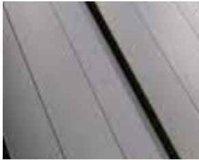
STANDING SEAM METAL ROOFING
