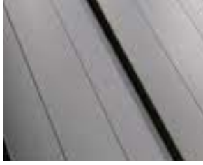
STANDING SEAM METAL ROOFING
