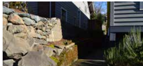
2. VIEW DOWN SOUTH PROP. LINE
