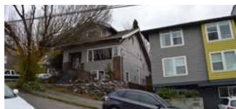
5. VIEW FROM ACROSS STREET
