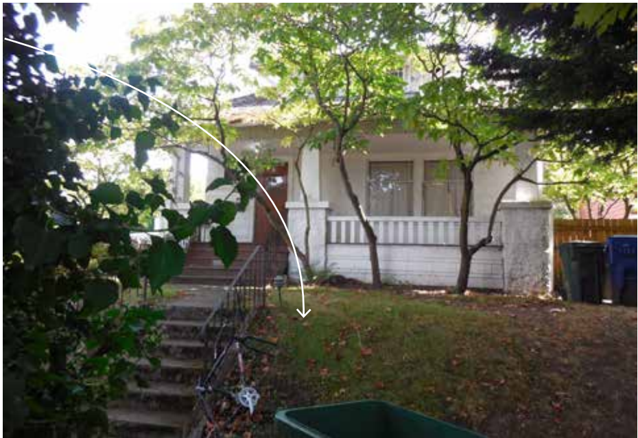
SITE CONDITION: RAISED GRADE AT NEIGHBOR
