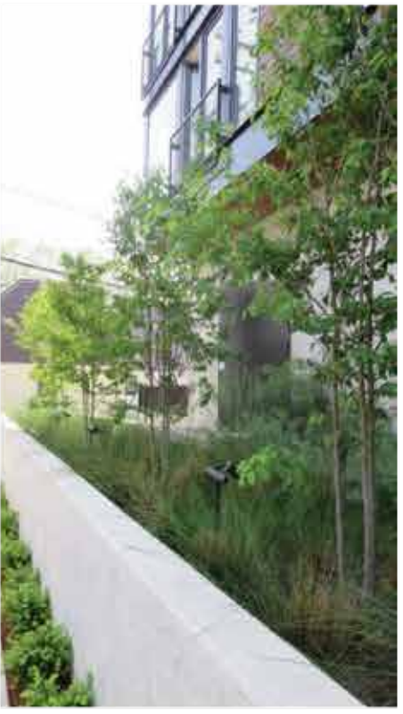
Bioretention Planter
