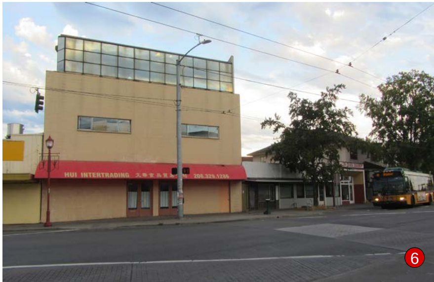
Commercial 3-Story Building Across From Site
