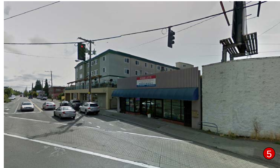
Commercial 1-Story Building South of Site, on 15th Ave S
