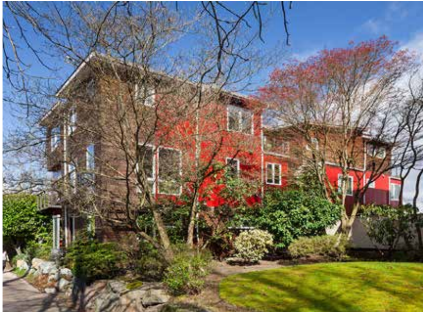
① 1530 15th Ave. E (View from sidewalk)
