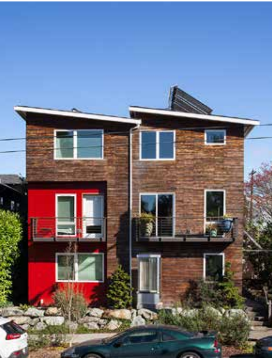
④ 1530 15th Ave. E. (View from street)
