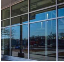
⑧ Storefront Glazing System -Aluminum, clear anodized finish
