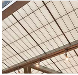
⑩ Kalwall Translucent fiber-reinforced polymer -translucent panels
