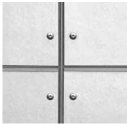
⑬ Fiber Cement Flat Siding -large format panels -metal reveals -color to match adjacent plank siding
