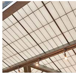
⑩ Kalwall Translucent fiber-reinforced polymer -translucent panels
