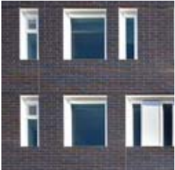
⑦ Vinyl Window System -white vinyl frame -recessed "shadow box" detail at openings
