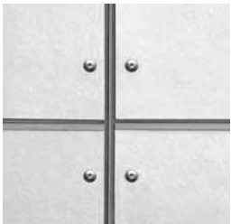
⑬ Fiber Cement Flat Siding -large format panels -metal reveals -color to match adjacent plank siding
