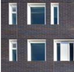
⑦ Vinyl Window System -white vinyl frame -recessed "shadow box" detail at openings
