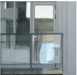
⑫ Glazed Guardrail System -42" transparent laminated glass with aluminum frame, painted "Silversmith".
