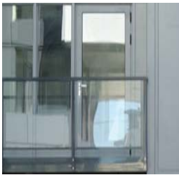
⑫ Glazed Guardrail System -42" transparent laminated glass with aluminum frame, painted "Silversmith".
