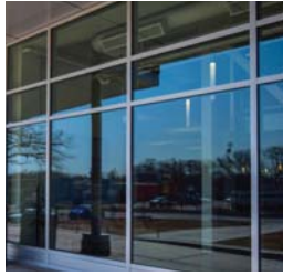
⑧ Storefront Glazing System -Aluminum, clear anodized finish
