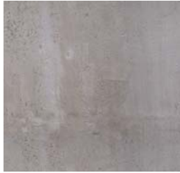
⑥ Cast-In-Place Concrete -light sandblasted architectural finish
