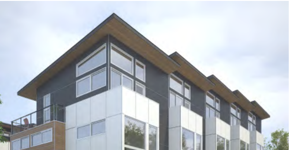
DC-2 and DC-4 Use of fiber cement of complementing colors, upper level setback, bay windows.
