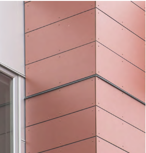
DC-4 Fiber cement wrapping of a corner
