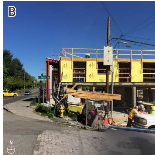
NEW MIXED-USE ACROSS FROM PROJECT SITE
