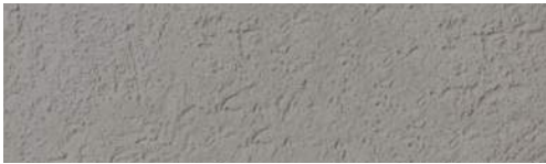
E. STUCCO & INSULATION OVER CONCRETE, GRAY FINISH
