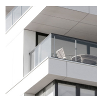
① Rainscreen Cladding System - 8mm thick through colored cement composite panels; matte finish; panel color "white" exposed fasteners to match
