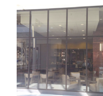
⑫ Storefront Glazing System - dark anodized finish mullions
