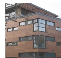
③ Rainscreen Cladding System - 10mm thk; phenolic panels; matte finish; exposed fasteners to match; walnut wood look or similar.
