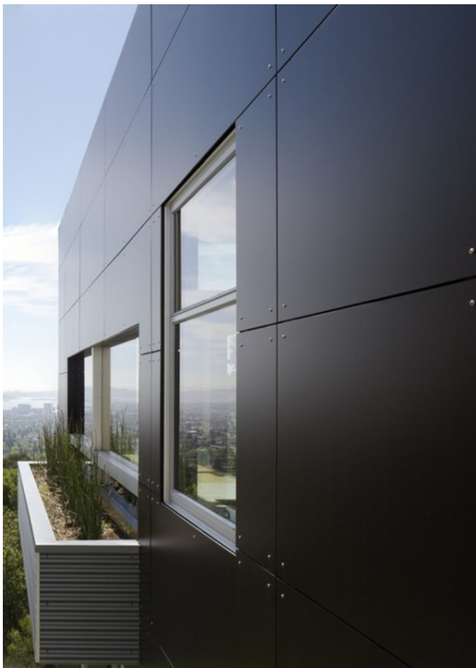
Hardie Panel Window Detail
