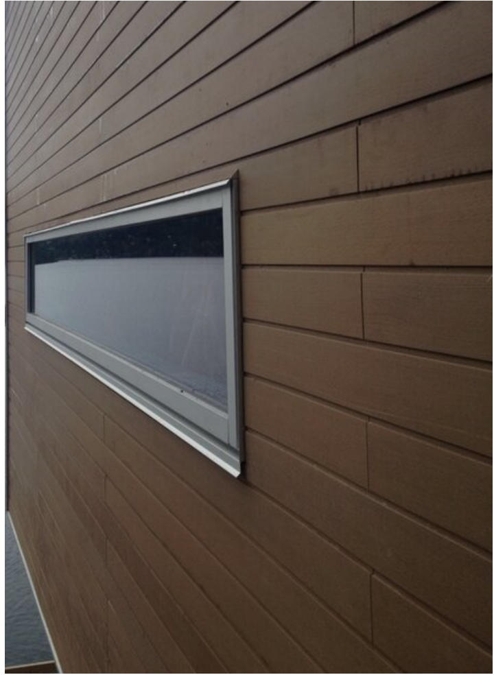
Window Trim at Resysta Siding
