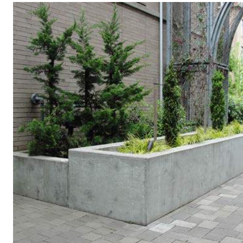
Integrated concrete planters
