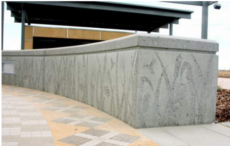
Concrete seat wall
