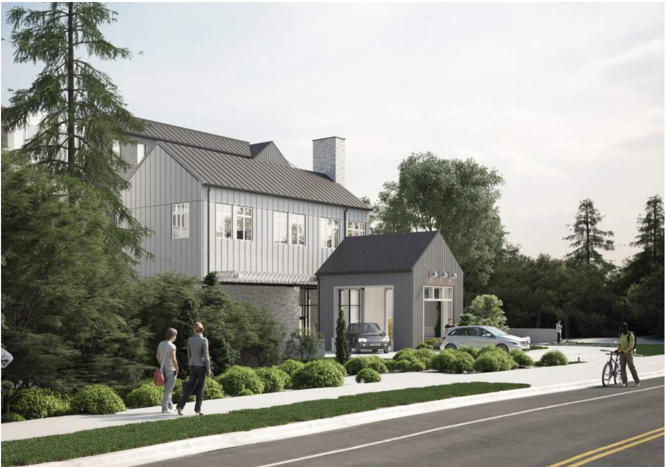
VIEW OF NORTHWEST CORNER
