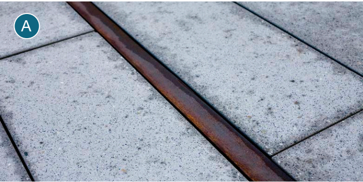
Precast Pavers and Steel Banding
