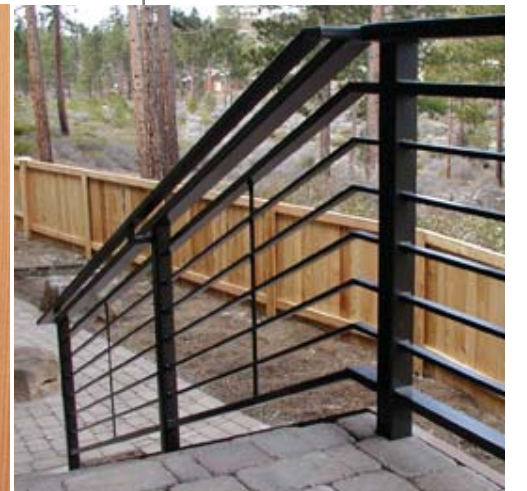
HORIZONTAL METAL RAILING PRECAST TREAD WITH WOOD STRINGER
