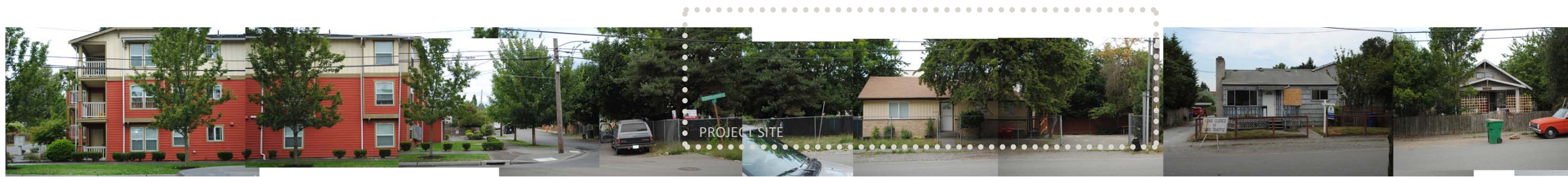
South Charlestown Street (looking North)
