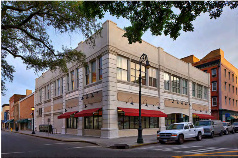
Retail Building - Savannah, GA
