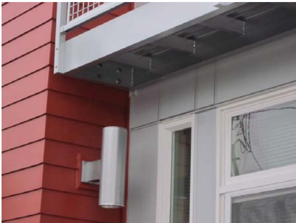
BOLT ON ATTACHED BALCONY
