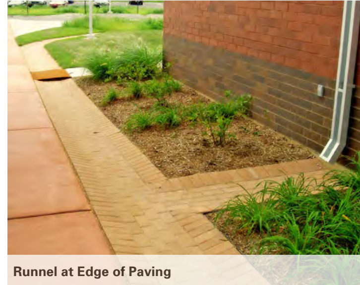
Runnel at Edge of Paving
