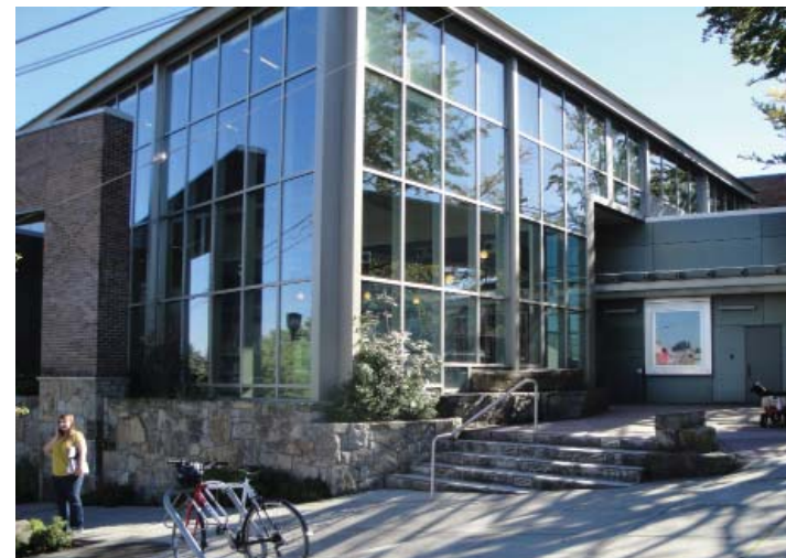
The (new) Greenwood Library on Greenwood Avenue
