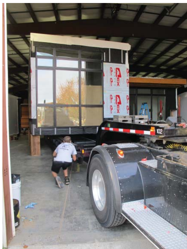
Controlled Construction Environment
