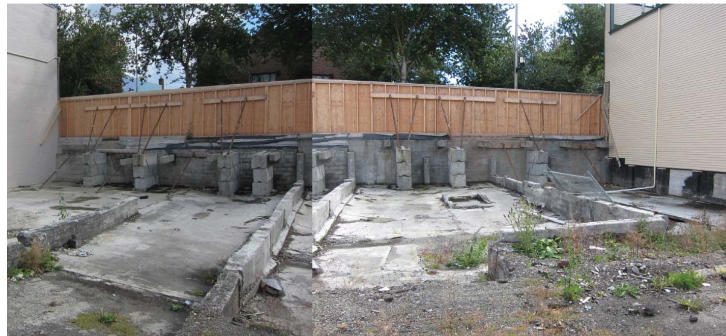
View of Site from North
