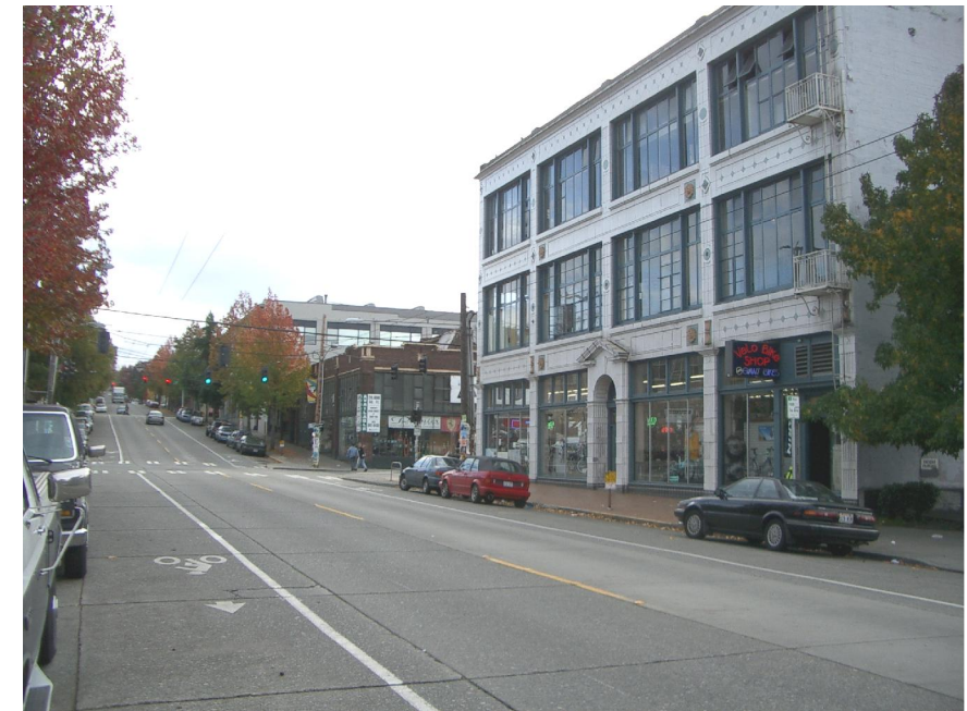
L. OLD REI BUILDING FROM PARK
