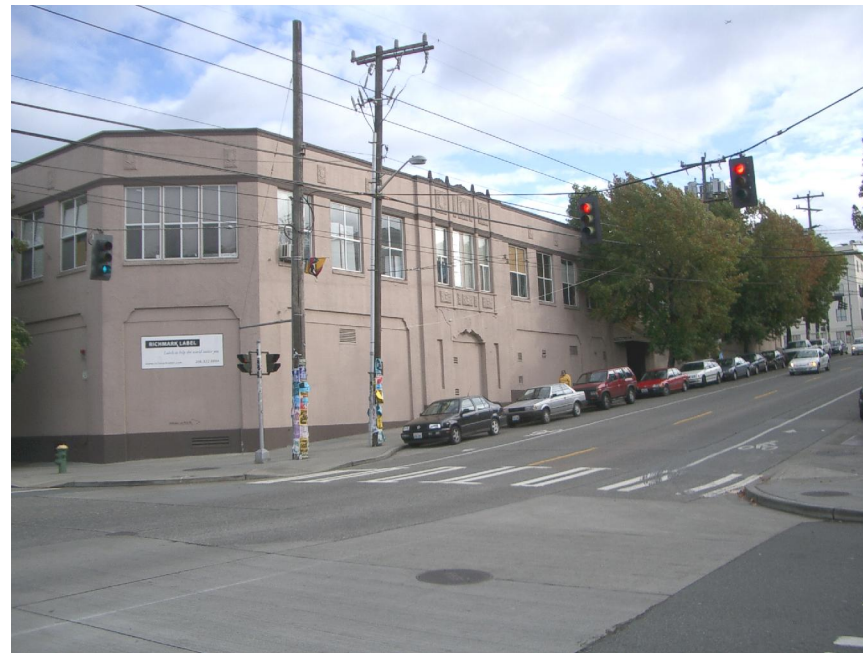
K. BLDG OCCUPIES THE ENTIRE BLOCK FROM 11TH TO 12TH
