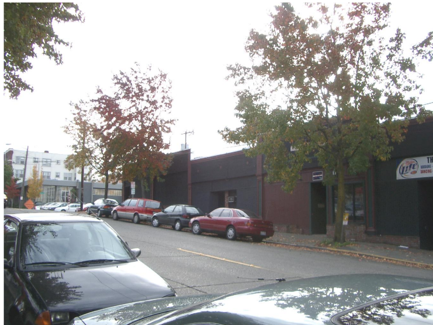
P. SOUTH SIDE. NO WINDOWS. PROBABLE FUTURE DEVELOPMENT
