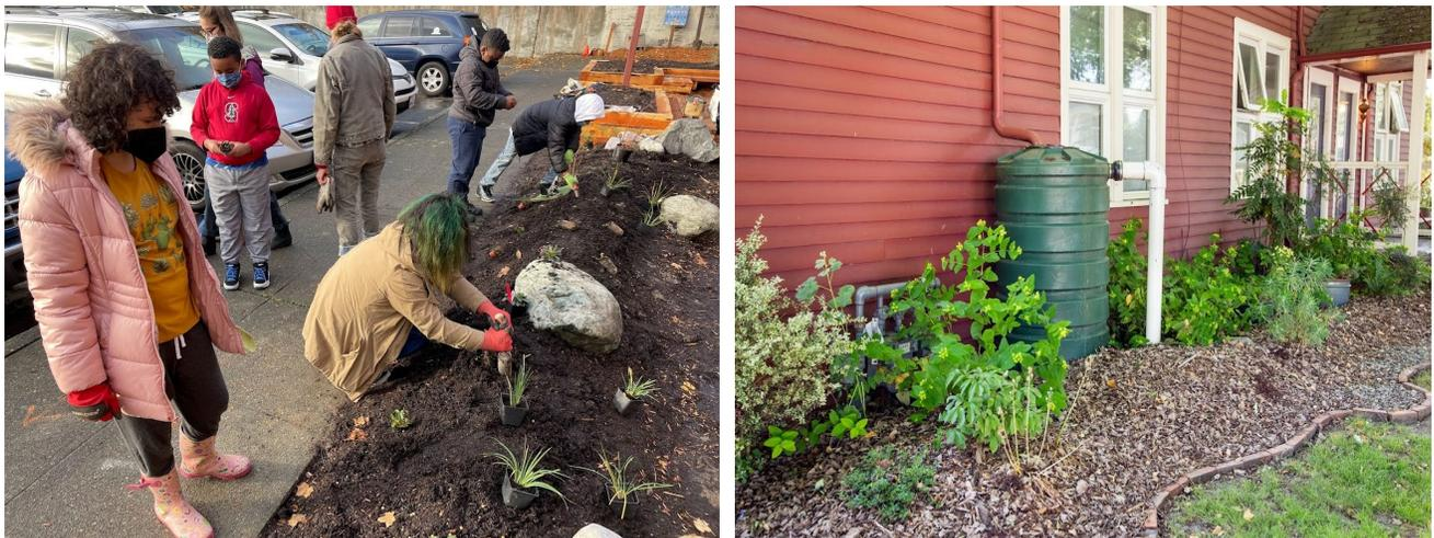
**Figure 4-8: RainWise school installation at Leschi Elementary (left) and typical cistern installation (right)**
