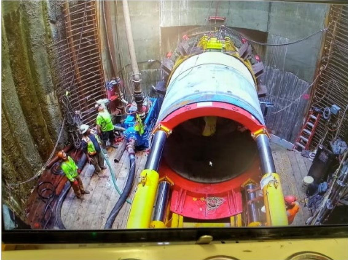
**Figure 4-6. 8 ft. Diameter Microtunnel Installation**
