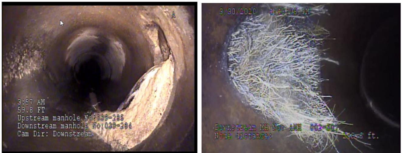
Figure 3-5. Private side sewer connections demonstrating visible FOG accumulations and impacts from root intrusion
