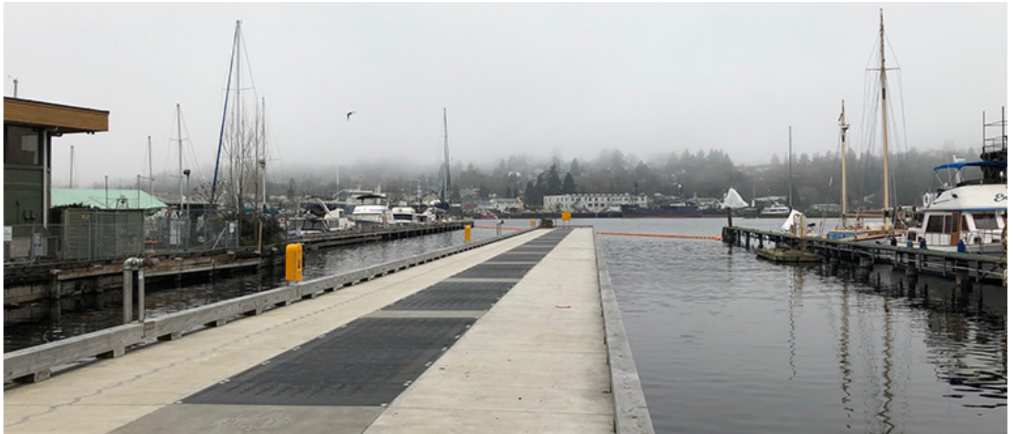
The reconstruction of the 24th Ave Pier was completed in 2019. The pier is open to the public.
