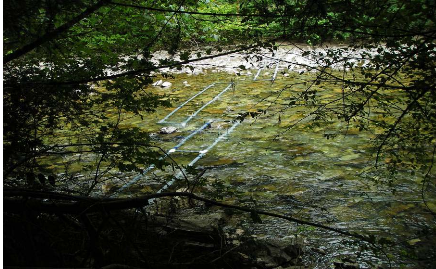
Figure 1.7.—Reinstallation of antennas 1, 2, and 3 in the Cedar River site, late August 2007. Antennas were placed in locations similar to those of the original installation, but larger fencing stakes were used as anchor points to secure the antennas.
