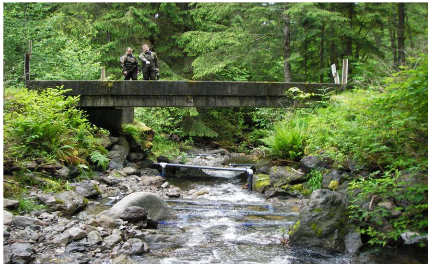
Figure 1.10.—Reinstallation of antennas 1, 2, 3, and 4 at Rack Creek, June 2006. Antennas 1 and 2, located upstream of the bridge, were pass-by antennas and antennas 3 and 4 were pass-through antennas. All were secured to the streambed by straps held to a combination of rebar stakes and anchor bolts in the substrate.
