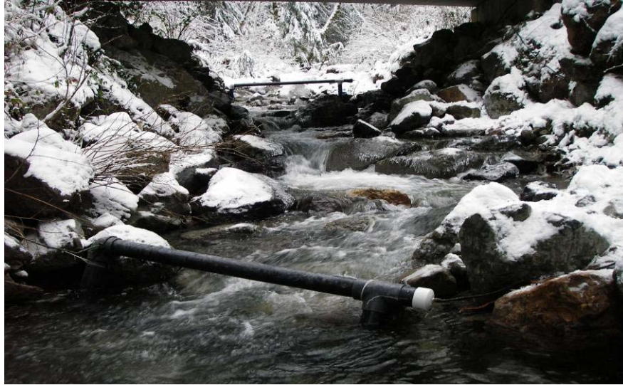
Figure 1.9.—Antenna array at Rack Creek following flooding that destroyed the array. The flooding occurred in early November and the antennas were reinstalled in late November, 2006. Antennas 1 (upstream) and 4 (downstream) were secured to anchor bolts in the substrate and were pass-through antennas.
