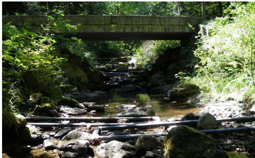
Figure 1.8.—Antenna array at Rack Creek, October 2005. Antennas 1 and 2, located under the bridge, were pass-through antennas and antennas 3 and 4 were pass-by antennas. All were secured to the streambed by straps held to a combination of rebar stakes and anchor bolts in the substrate.
