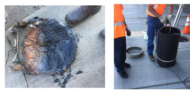
Figure 4-1. Removed Flap Gate (left) and New Backwater Valve (right) in Basin 107
