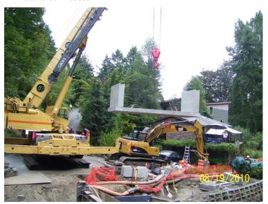
**Tip:** Where staging is limited and/or the project is linear, with some parts a significant distance from the staging area, consider designing with materials that can be installed or worked out of a dump truck. For example, because of staging limitations it may be more cost effective to haul out all excavated material and to backfill with imported material. Controlled density fill (CDF) placement requires the least amount of equipment.
