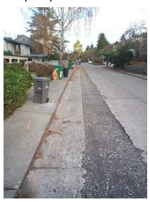
**Tip:** Understand how temporary pavement edges will tie into existing pavement and castings. In some cases, the best approach may be a hybrid of materials such as Permanent base AC with cold mix at the edges. Sometimes the decision is best made as a field adjustment. If a field adjustment is planned, discuss the bid items needed with the construction management supervisor on the project.
