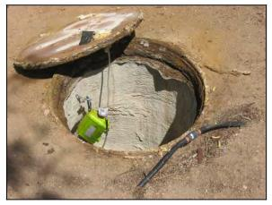
Figure A-5. Installed Pressure Monitor
