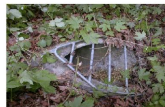
Overflow Level Grated Inlet to MH (Pond Outlet)
