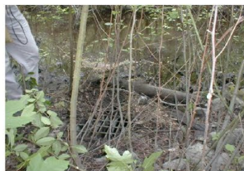
Low Level Grated Inlet to MH (Pond Outlet)
