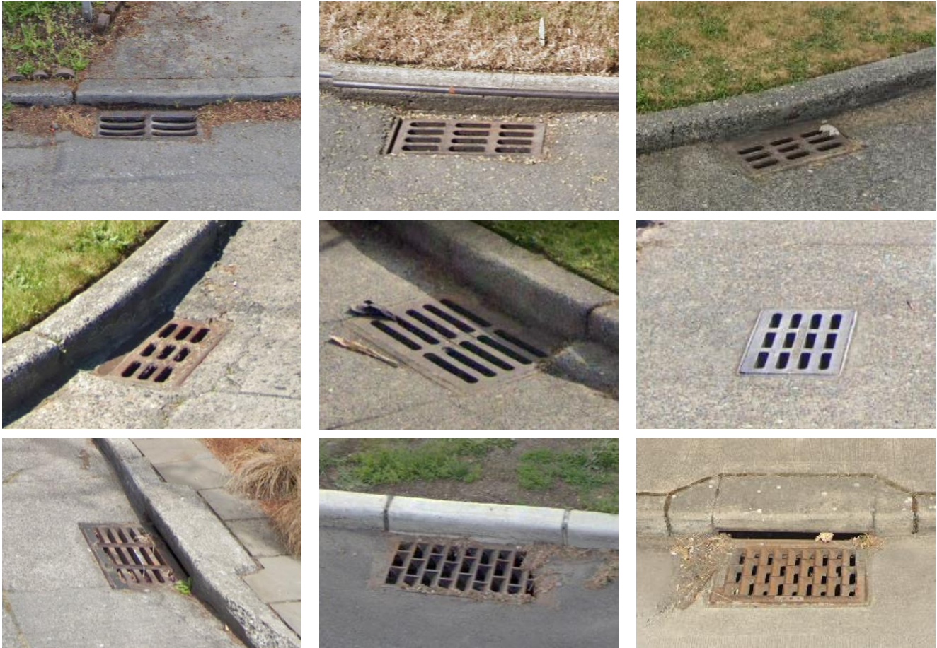
Figure 3-8. Examples of different inlets to SPU collection systems
