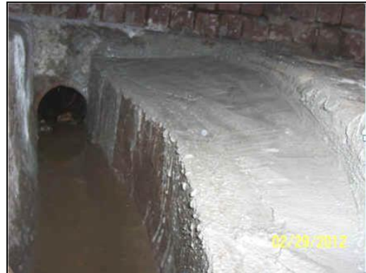
Figure 2: S Brighton CSO after sealing.
