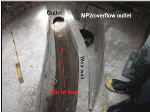
Figure 1: S Brighton CSO before sealing.
