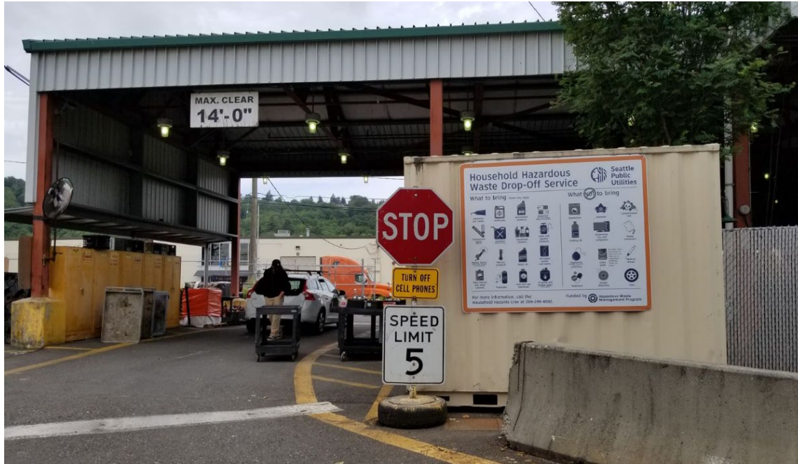
The South Household Hazardous Waste Facility drop-off (Source: Hazardous Waste Management Program)
