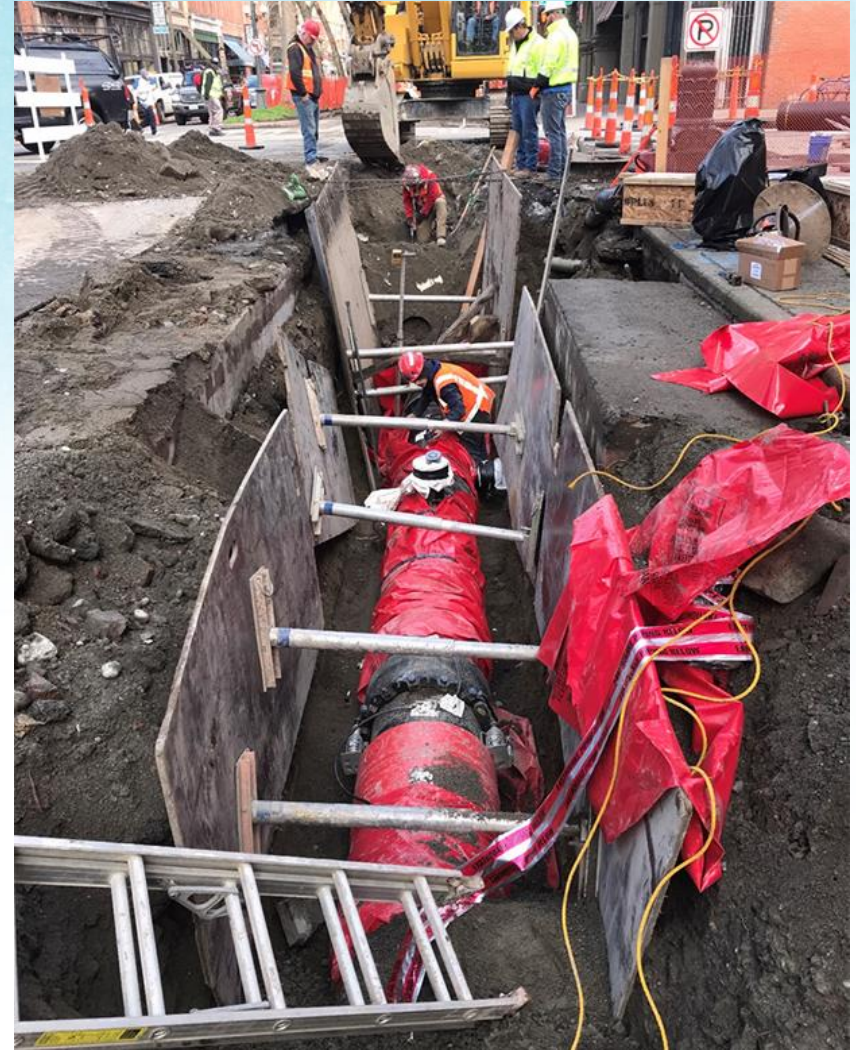
Earthquake resistant pipe installation in Pioneer Square
