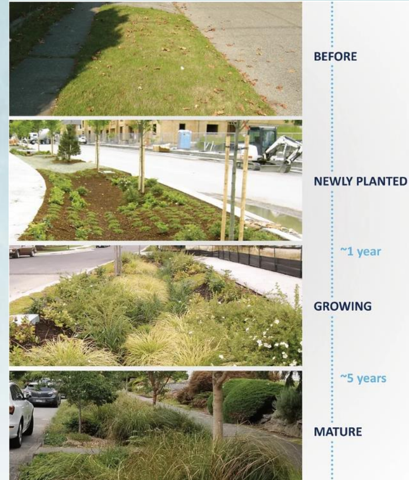
How a typical NDS planting installation changes over time
