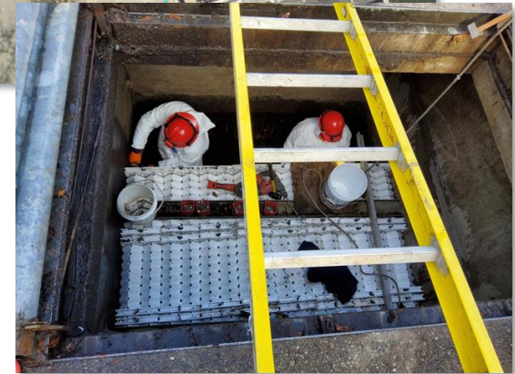
Drainage Facility improvements photos, replacing of plates of an Oil/Water Separator at Green Lake
